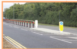
Street signs/bollard lights
