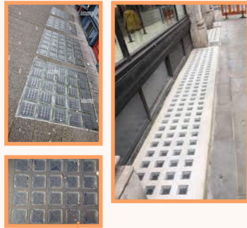
Skylights/pavement lights (potential basements)
