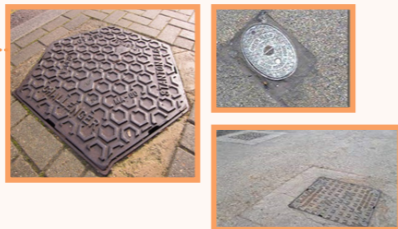
Manholes/ducts/access covers/drainage rodding points
