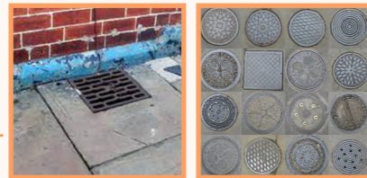
Coal chutes, hatches (potential basement) and vents
