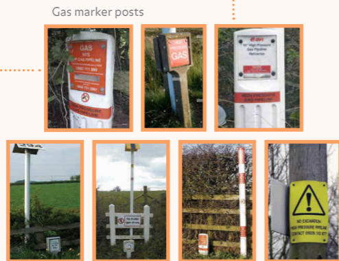
Gas marker posts
